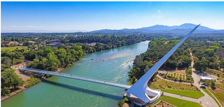
*The Sundial Bridge is a cantilever spar cable stayed bridge for bicycles and pedestrians that spans the Sacramento River in Redding and forms a large working sundial.*
